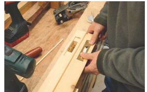
▲ Pic.6 Sash pulleys are mortised into the stiles as shown
